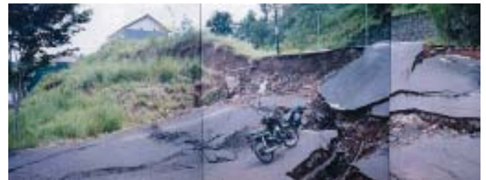
Figure 2: Damages due to subsidence
