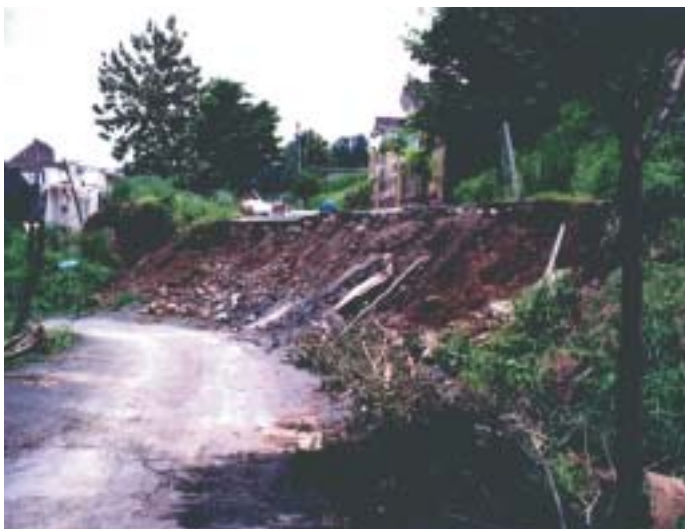
Figure 5: Land subsidence causing different elevation
