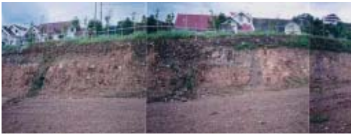
Figure 1: Excavation in the breccia layer
