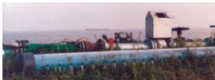
Figure 4: Close-up of the experimental setup for generating the constant 'overtopping' flow rate of 1 l/s over a stretch of thirty meters
