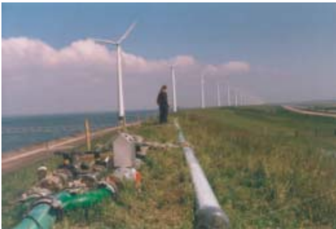
Figure 1: IJsselmeerdijk, including the experimental setup on top of the crown of the waterretaining structure. The inner slope is to the right hand side, the fence on the right of the picture is placed on the intermediate shoulder.
